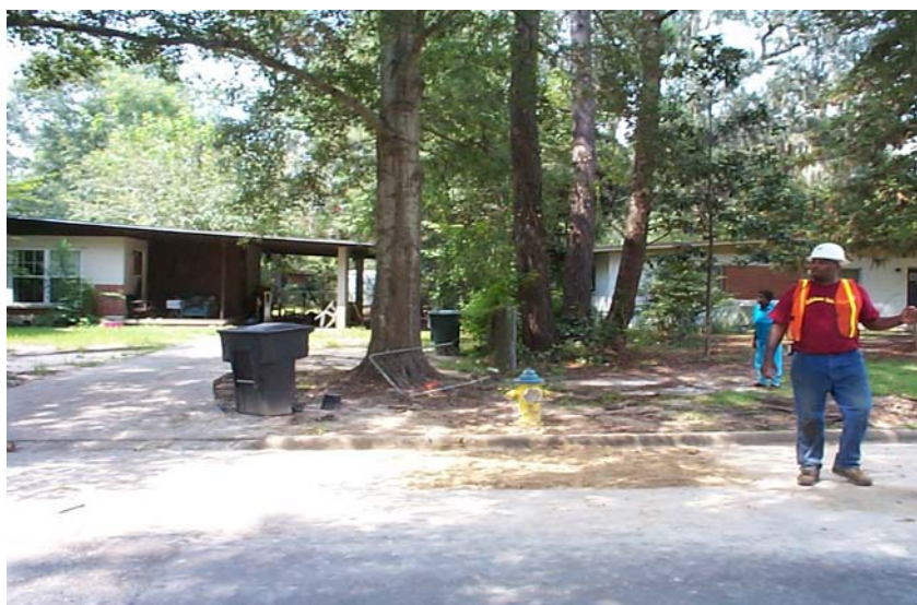
City workers install a new fire hydrant in the neighborhood
